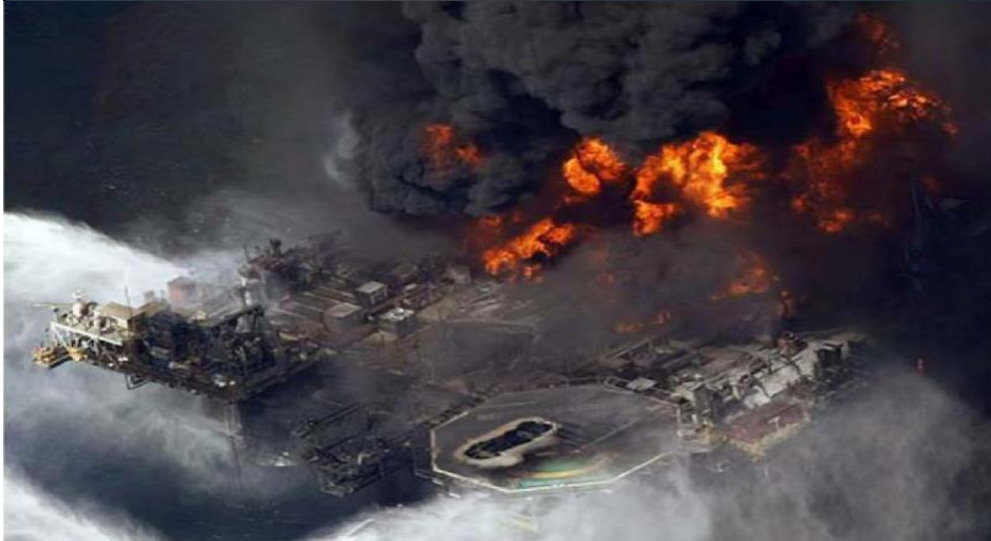
Early morning Day 2 – Note the hole burned through the aluminum helideck
